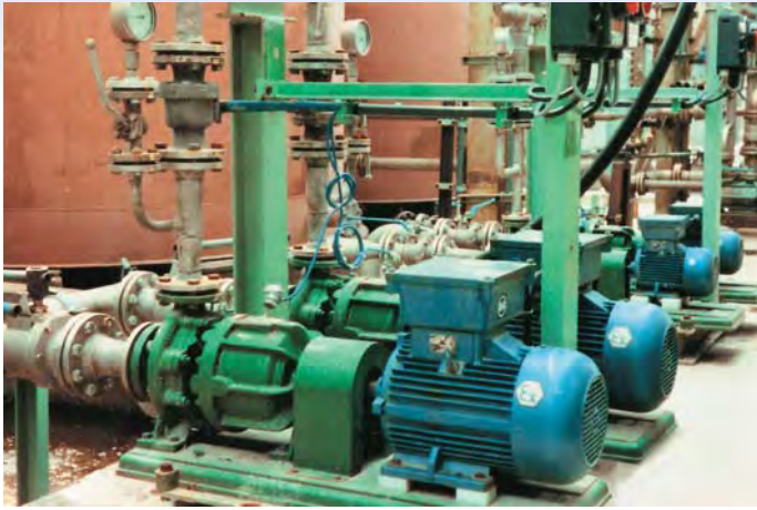
Type NML with magnetic coupling. Liquid: Methylene Chloride, 40°C (104°F).
