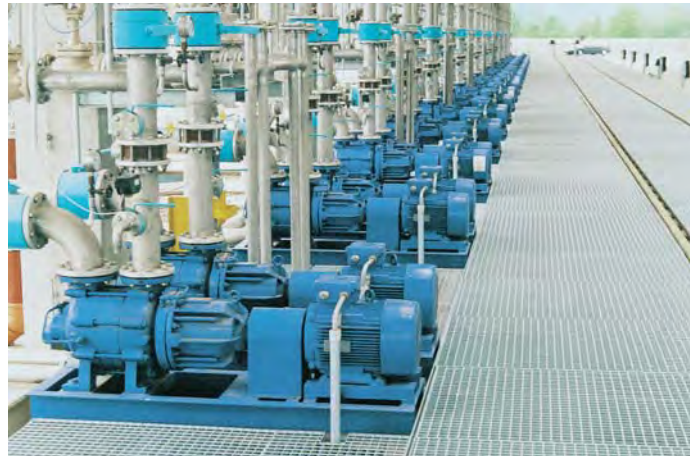
Type HZSM with magnetic coupling. Liquid: Solvent, 20°C (68°F).
