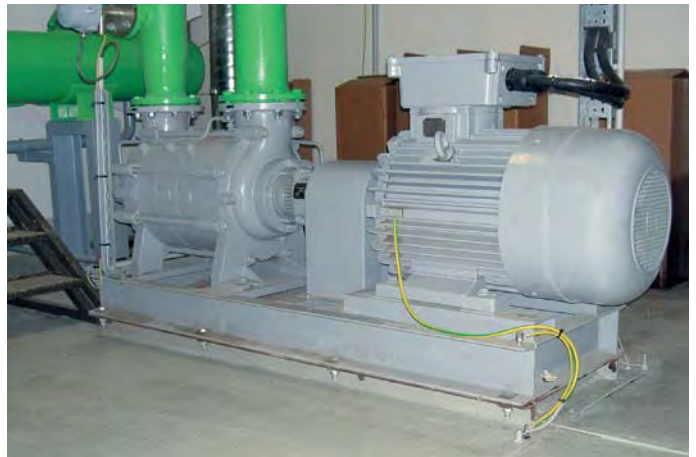
Type HZS with single mechanical seal. Liquid: Gasoline, Diesel 20°C (68°F).
