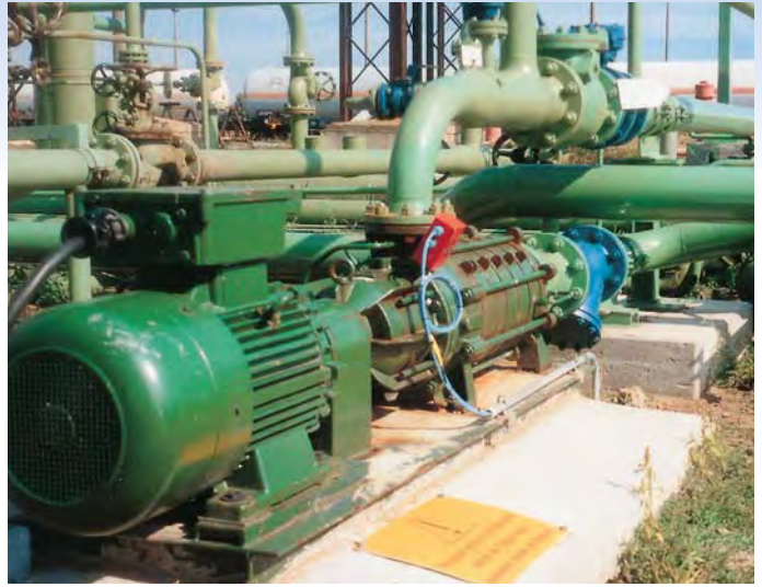
Type HZSMA with magnetic coupling. Liquid: Propane/Butane, 20°C (68°F).
