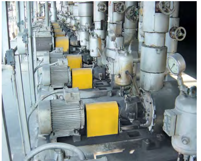
Type NCL with tandem bellows seal (N9). Liquid: Thermal oil, 330°C (626°F).
