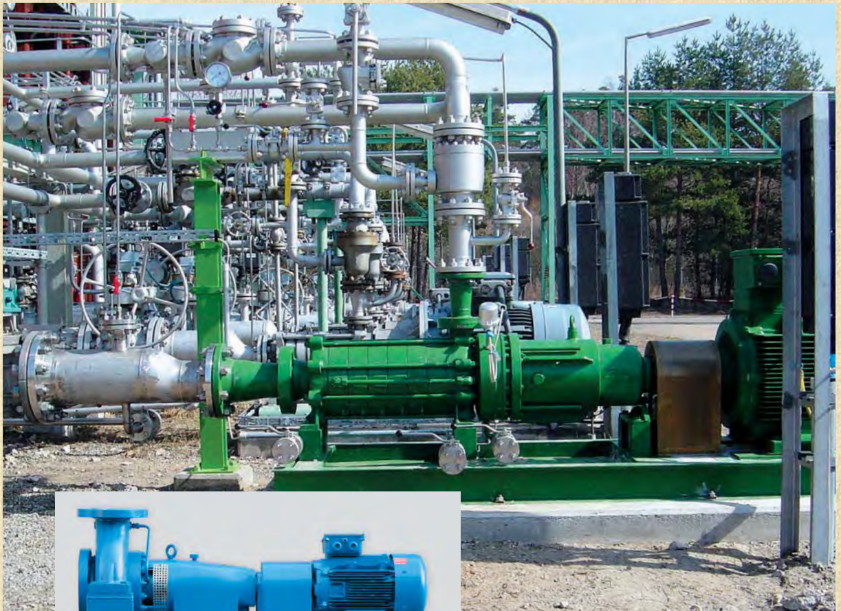
Type PRM with magnetic coupling 275 kW. Liquid: Chlorosilane 116°C. Design pressure 35 bar/150°C
