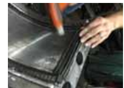
Installing the circumferential and longitudinal packing
