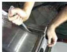
Relieving the GirderRing
