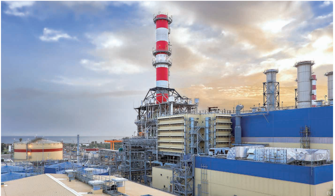
Large-scale power plant
