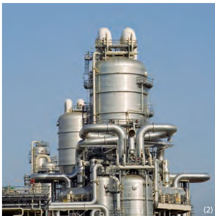
Chemical process combustion
